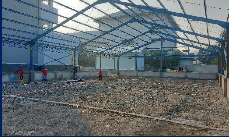
Erection Steel Structure Daito Cevest
