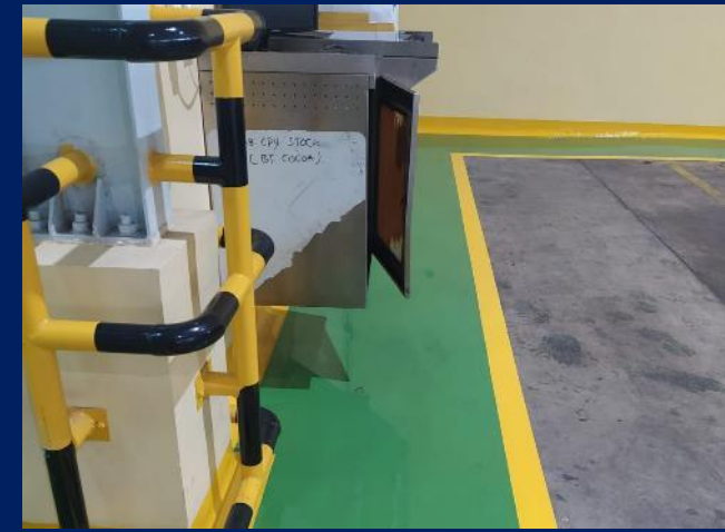
Epoxy Floor Warehouse
