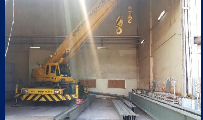
Erection Steel Structure Olam Cocoa
