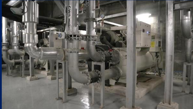
Water Cooled Screw Chiller
