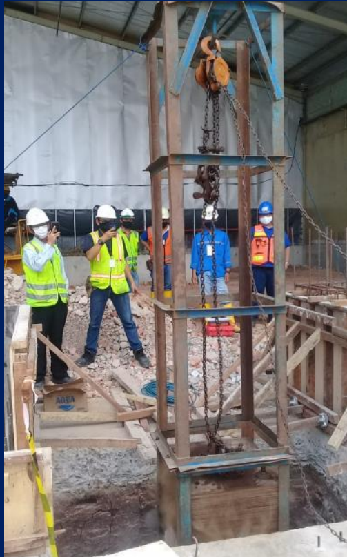
PDA Test Tiang Borepile
