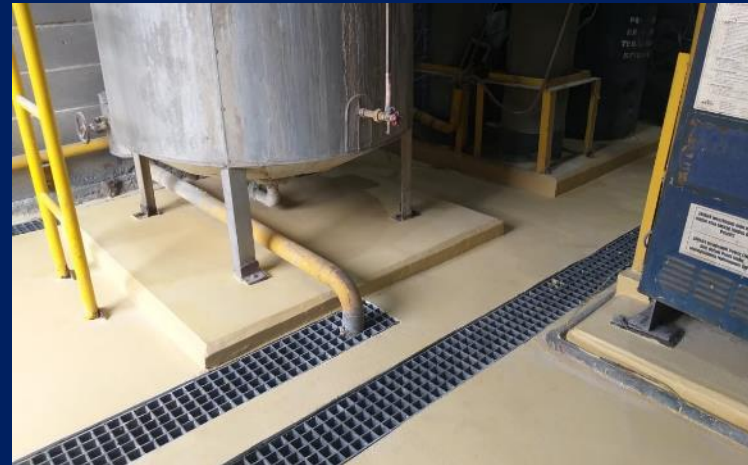
PU Flooring Boiler Room
