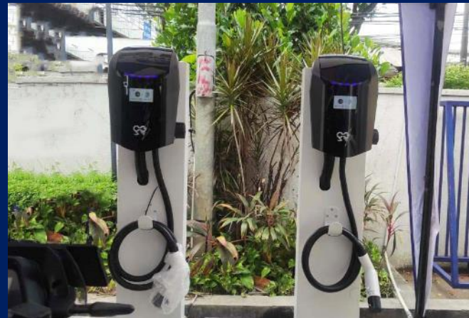
Installation Works for Motorcycle
