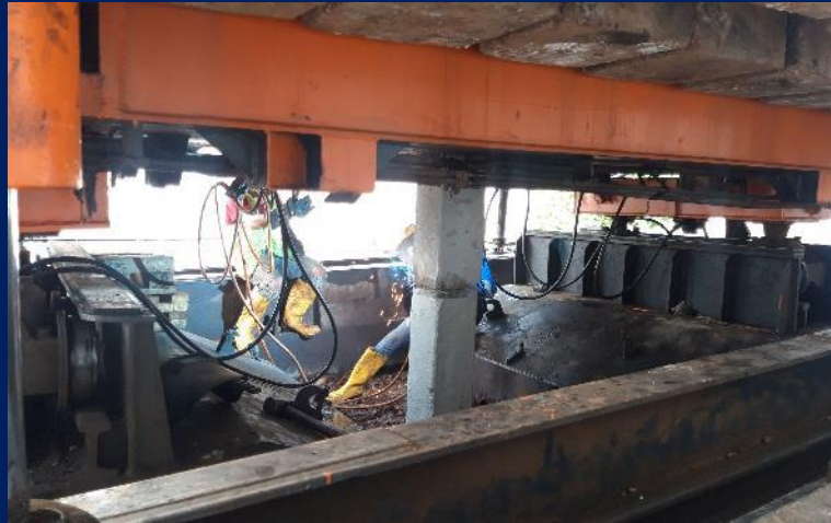
Join Pile Tiang Pancang
