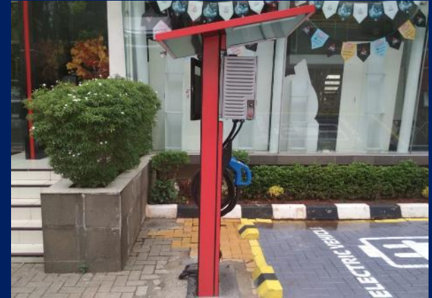
Installation Works for Car
