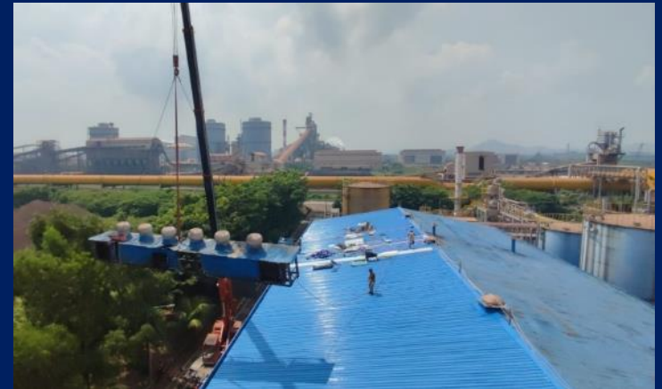
Demolish Roof Fan
