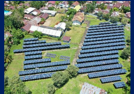
Energy Management System Sumba Island - NTT
