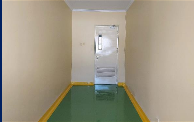
Epoxy Floor Office
