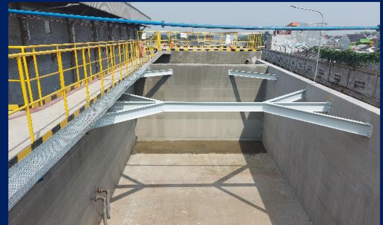
Gutter U Ditch WWTP
