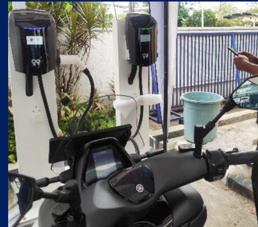
Installation Works for Motorcycle
