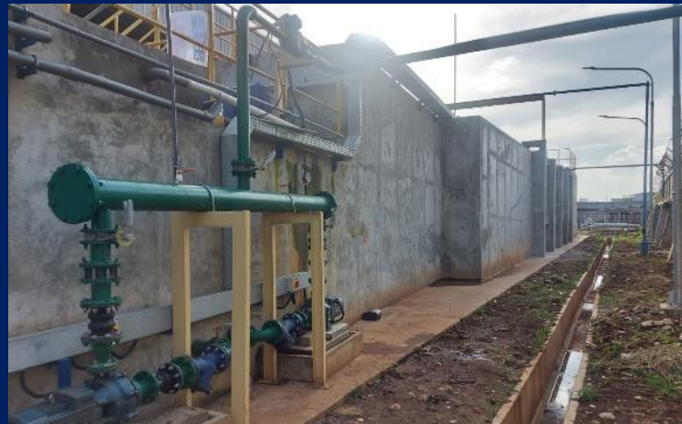
Gutter U Ditch WWTP
