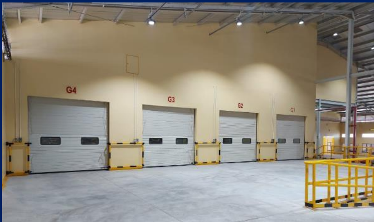
Loading Bay - Warehouse
