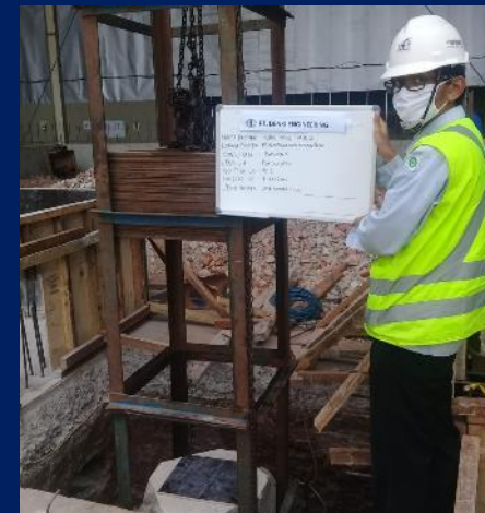
Persiapan PDA Test Tiang Borepile
