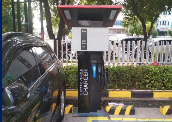
Installation Works for Car
